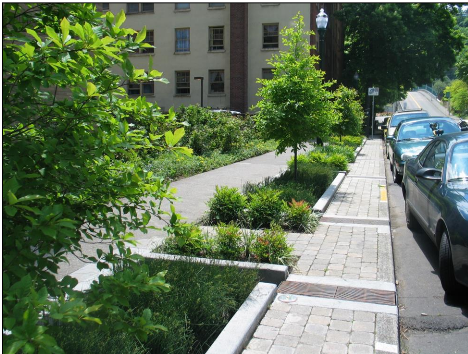
EXAMPLE OF BIOSWALE AND PERVIOUS PAVEMENT
