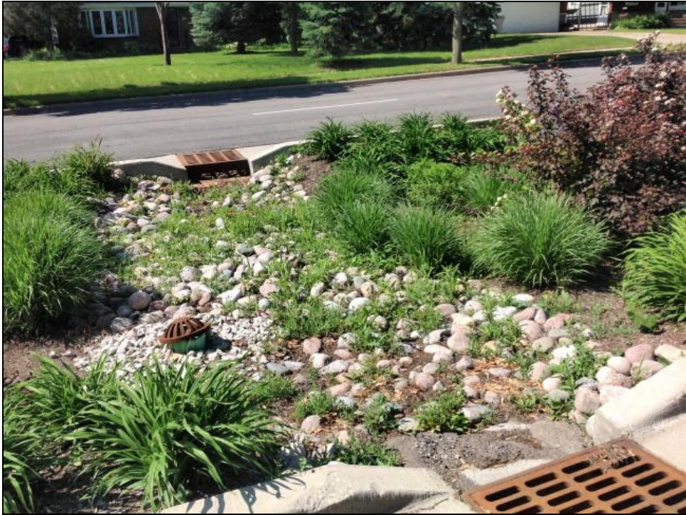
EXAMPLE OF BIORETENTION
