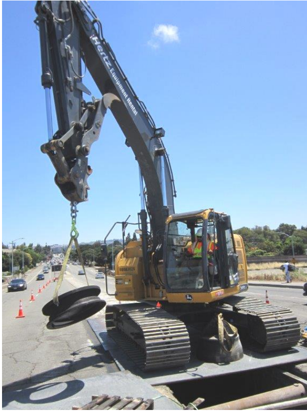
A rented excavator being used to repair a utility pipeline.
