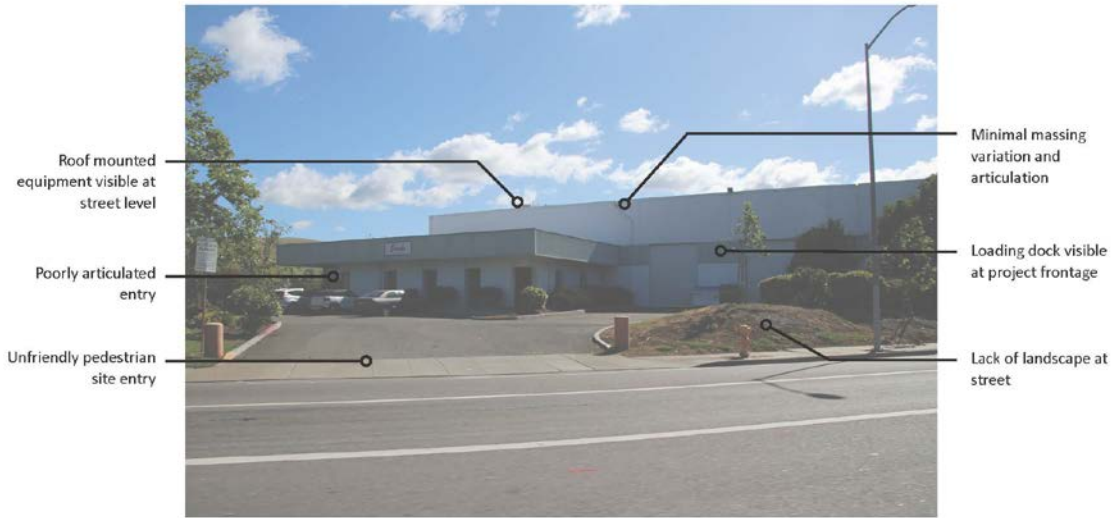
Older industrial development typically exhibit a lack of landscaping, recessed or less articulated entries, loading docks in the front or near the street, and minimal employee amenities
