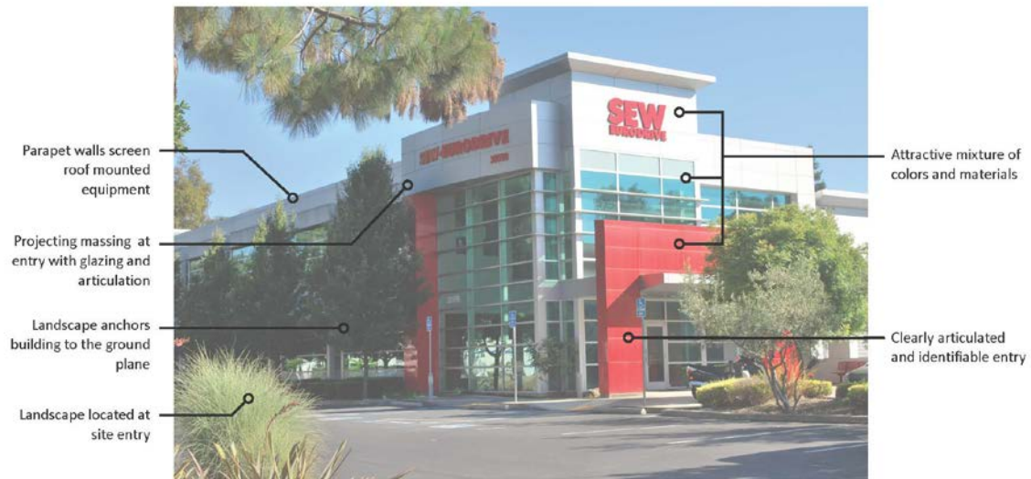
Recent industrial developments reflect current design trend characteristics; such as coordinated landscaping along frontages, prominent entries with articulation and detailing, loading docks at the side or in the rear, and employee amenities, among others
