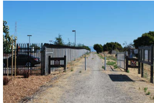
The requirement for landscaping adjacent to the Bay Trail, is vague and not been consistently implemented.
