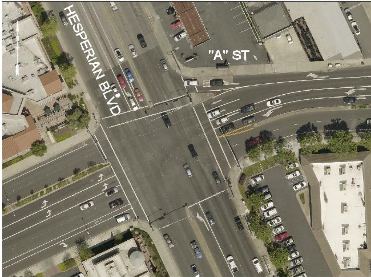
Figure 1: A Street and Hesperian Boulevard Existing Conditions
