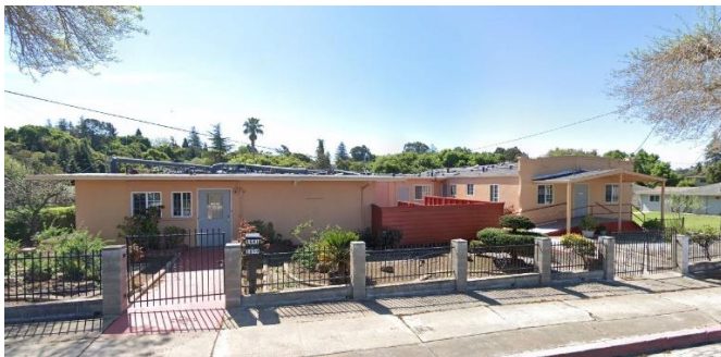
Building #1 (1659 D St.)
