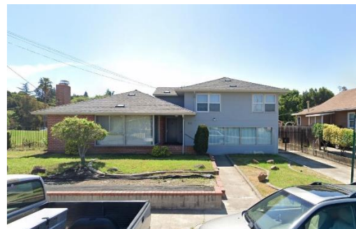
Building #2 (1641 D St.)
