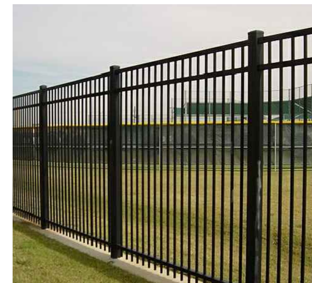
TUBE STEEL VIEW FENCE
