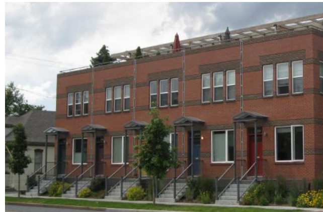
Stoops define the entries to this Rowhouse building while elevating the ground floor from the street level.
