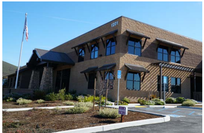
Articulation and detailing continue on side elevation through use of windows, awnings, and other detailing.
