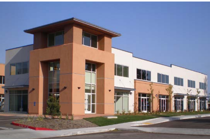
Window proportions complement architectural style and clerestory windows are used to allow interior natural daylighting.
