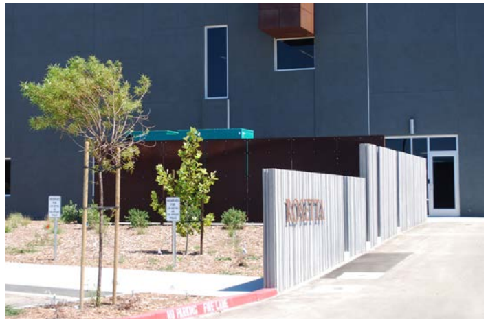
Wall and fencing designed as integral part of a site through continuation of building materials, with landscape minimizing visual monotony.
