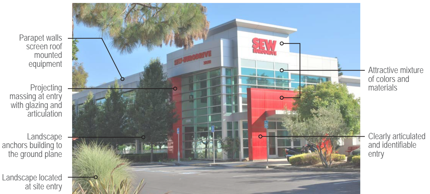
Example of recent industrial development reflecting current design characteristics.
