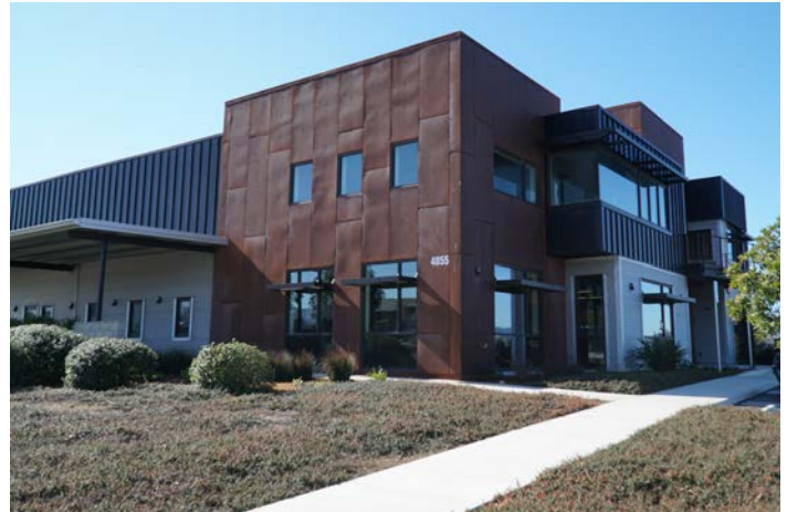
Pedestrian pathways are easily identifiable and connect the building to parking areas and off-site sidewalks.
