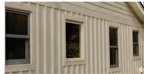
2 VERTICAL SIDING FIBER CEMENT BOARD AND BATTEN
