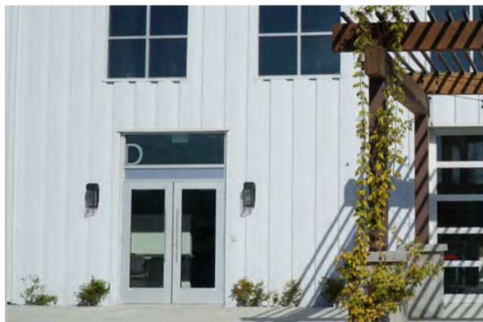
Light fixtures mounted at appropriate height for setting adjacent to building entry and shielded downward.
