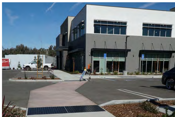
Unique, colored paving clearly identifies pedestrian pathway through parking area.
