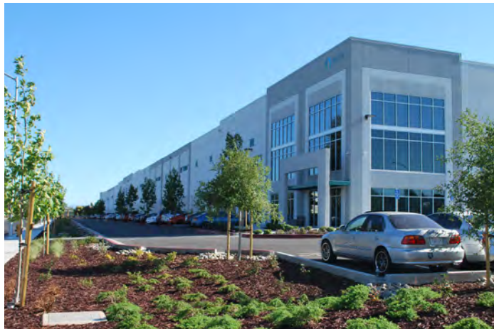
Street facing building elevation includes variation in wall plane, wall height, and roofs at different levels.
