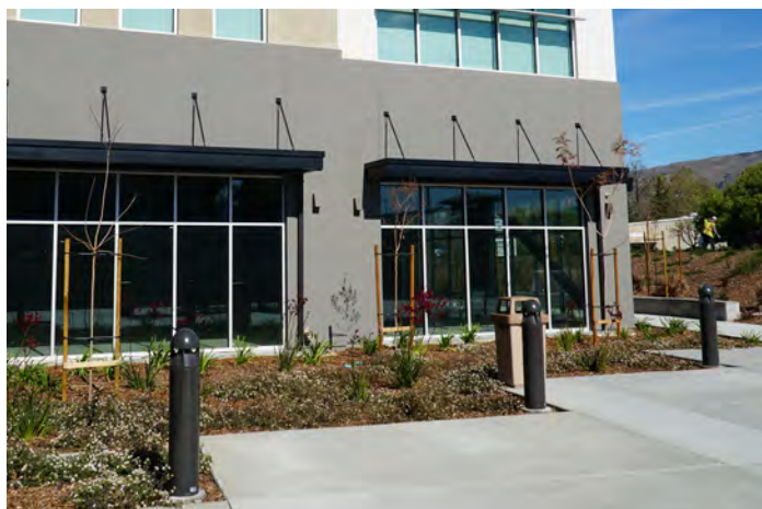
Low, bollard light fixtures placed to provide lighting within pedestrian areas.
