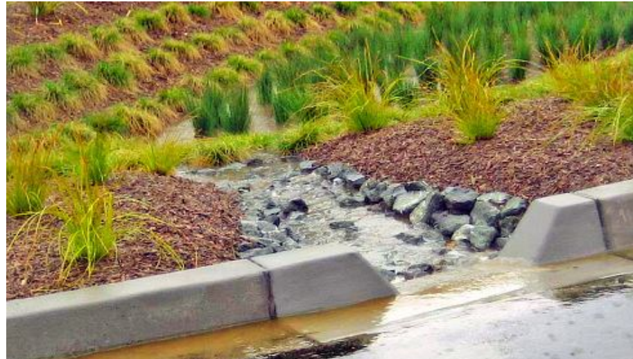
CURB CUT + BIOSWALE
