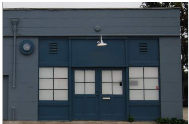
Maker Shopfront with double doors for each entry.
