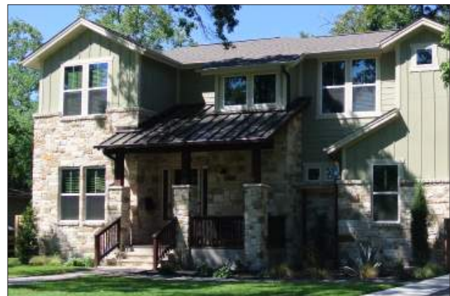
A projecting porch on the front facade that creates a nice seating space.
