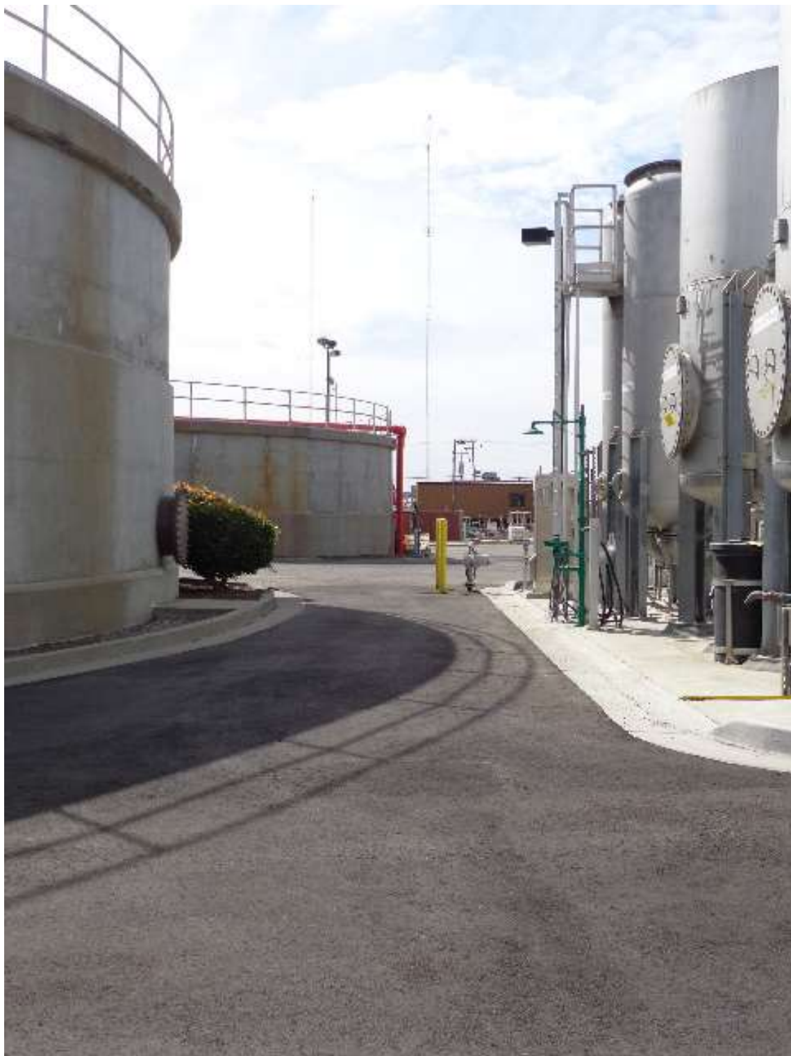
Access on East Side of Vessels
