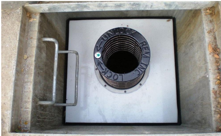
Figure 3: Small Trash Capture Device within Storm Drain
