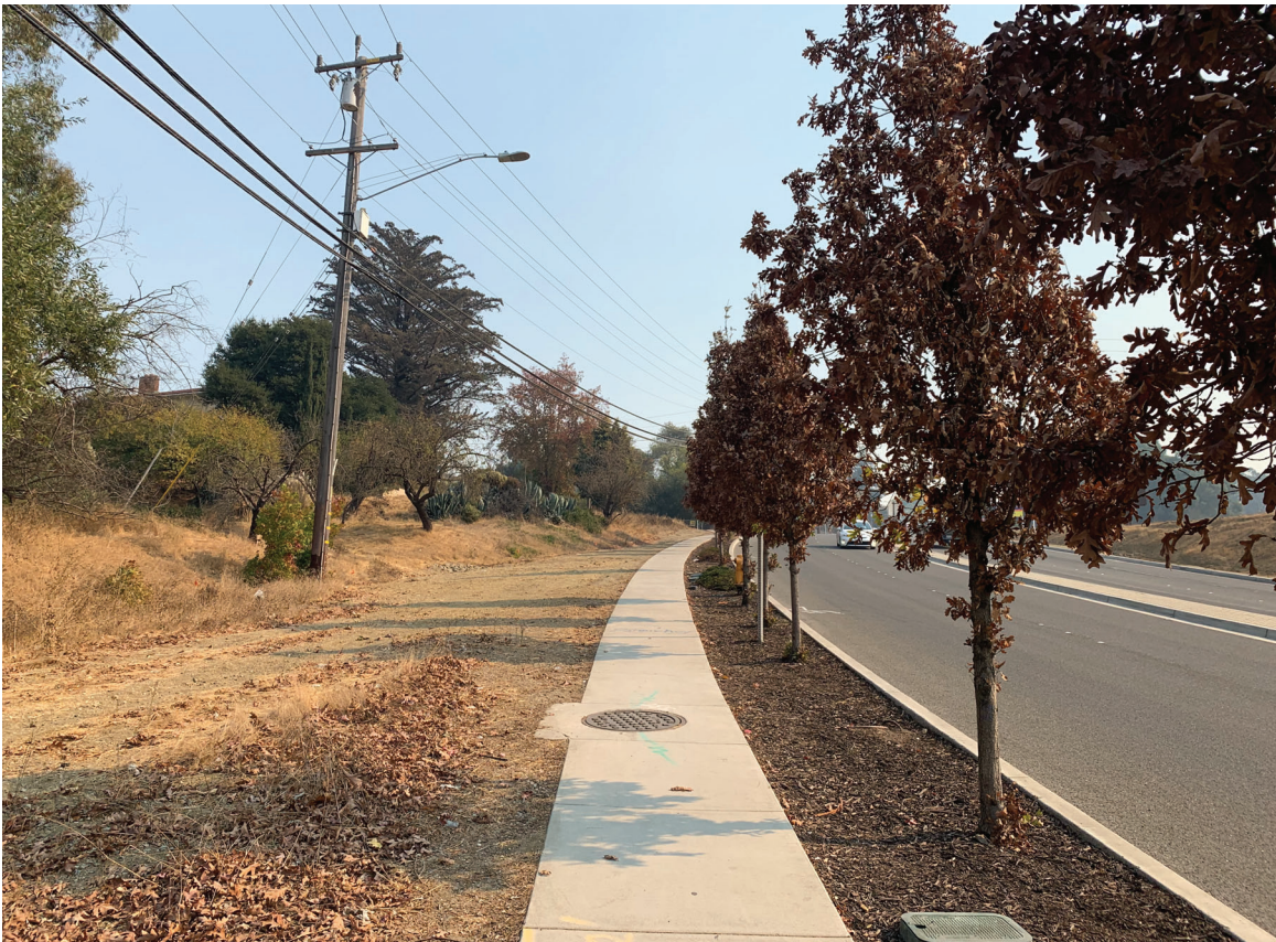
Photo 2: View of the project site from the west along Carlos Bee Boulevard.
