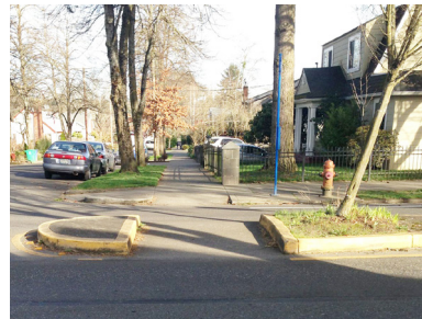
Raised median at refuge with clear waiting area for pedestrians crossing the street
