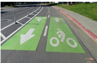
Cycle track pavement markings
