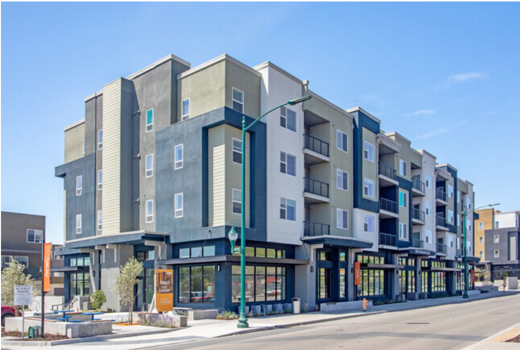
The Mix / Hayward, CA. Building height to the highest roof plane is 46' for 4 stories and to the highest parapet is 55'
