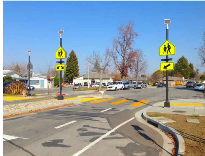
Rectangular Rapid Flashing Beacons (RRFBs)
