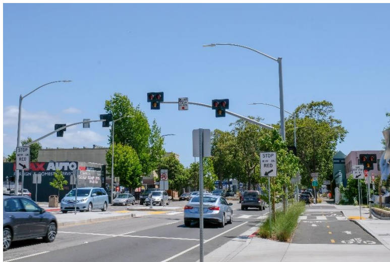
Pedestrian hybrid beacons provide better safety and comfort for pedestrians crossing, especially at high-volume and high-speed roadways Source: Kittelson & Associates, Inc
