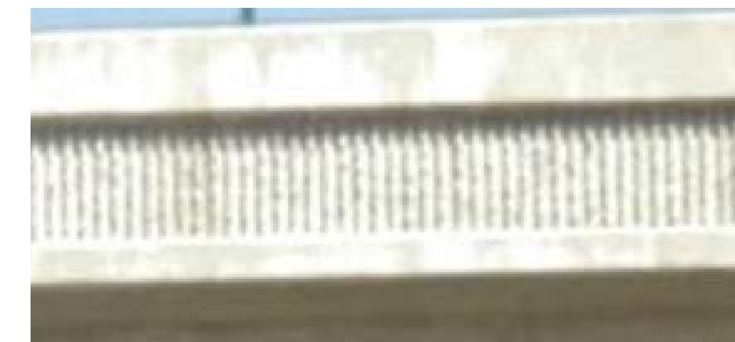
CONCRETE BARRIER INSPIRATION
