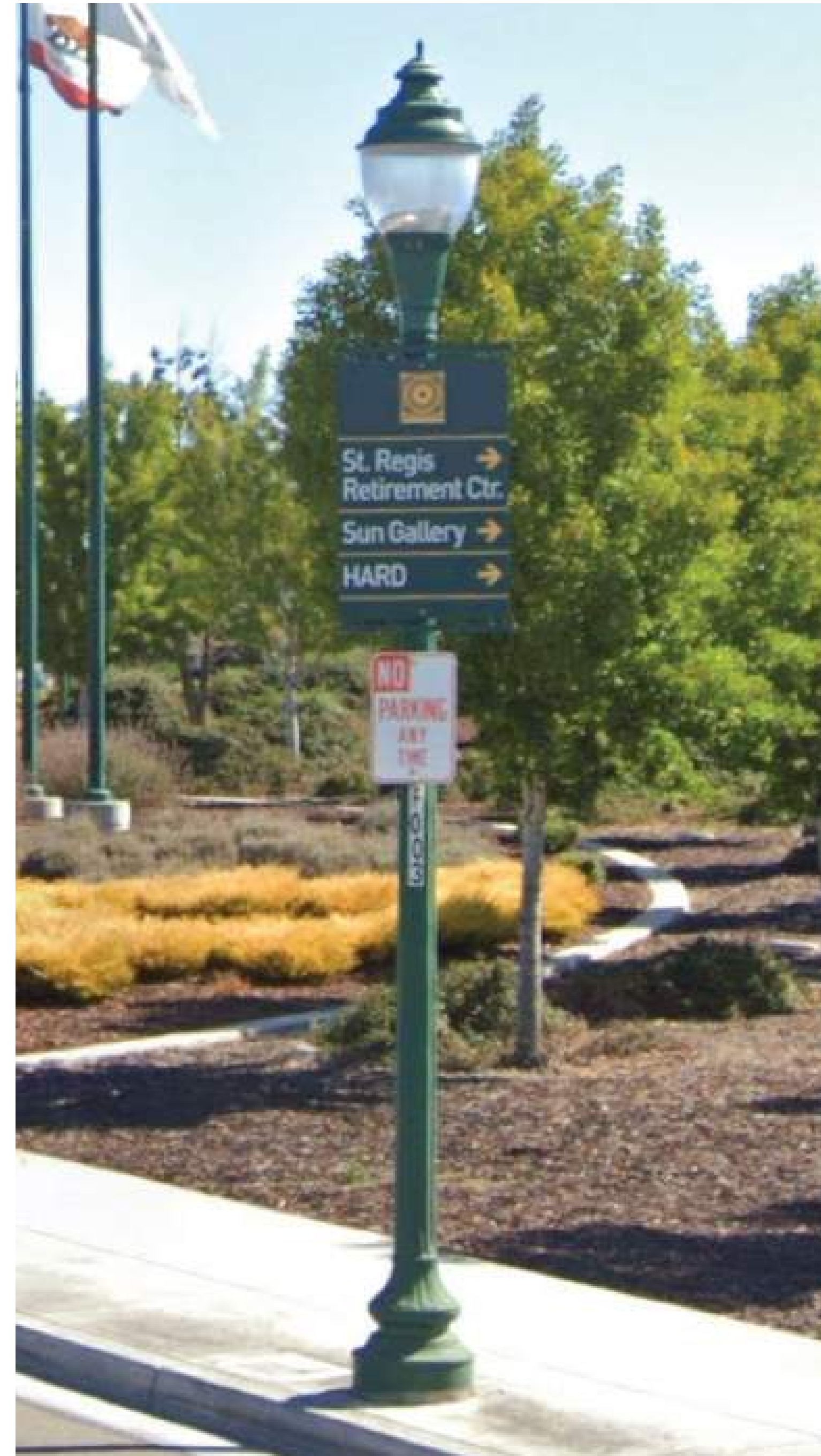
CITY OF HAYWARD PEDESTRIAN POLE LIGHTING WITH WAYFINDING SIGNAGE
