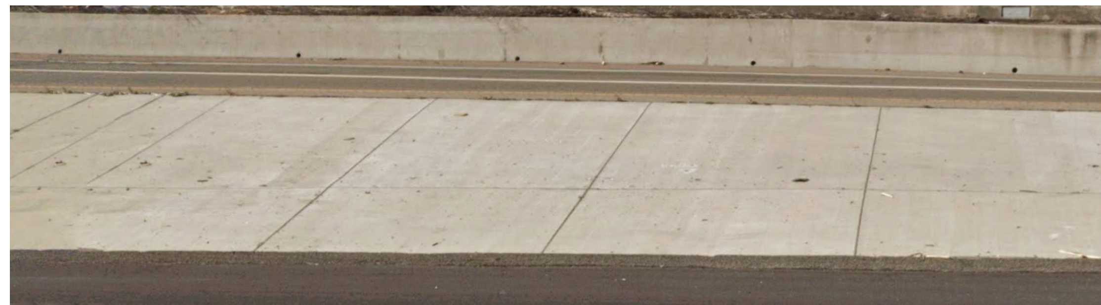
GORE PAVING AT 92/880 INTERCHANGE
