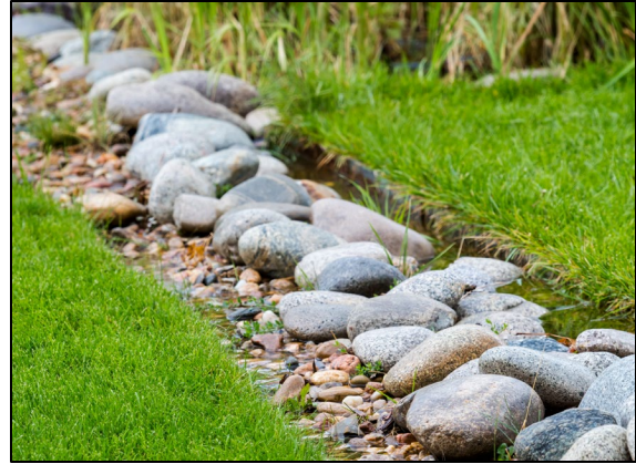
Figure B-9. Pervious Drainage Channel. Pervious, unlined drainage channels can be designed to convey runoff to GI facilities.
