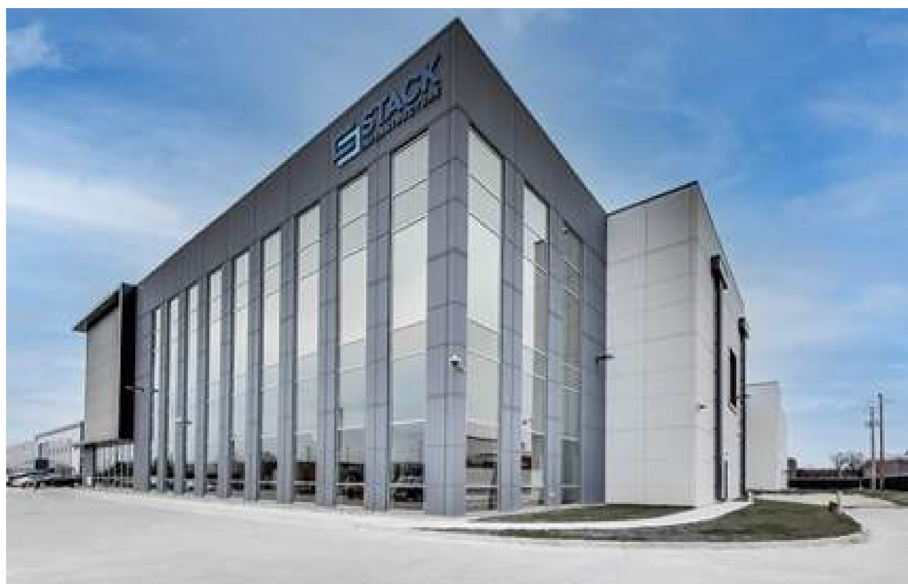
MATERIALS: METAL PANELS, CONC PANELS GLAZING: SPANDREL, TINTED COLORS: SILVER, WHITE, DARK ACCENTS
