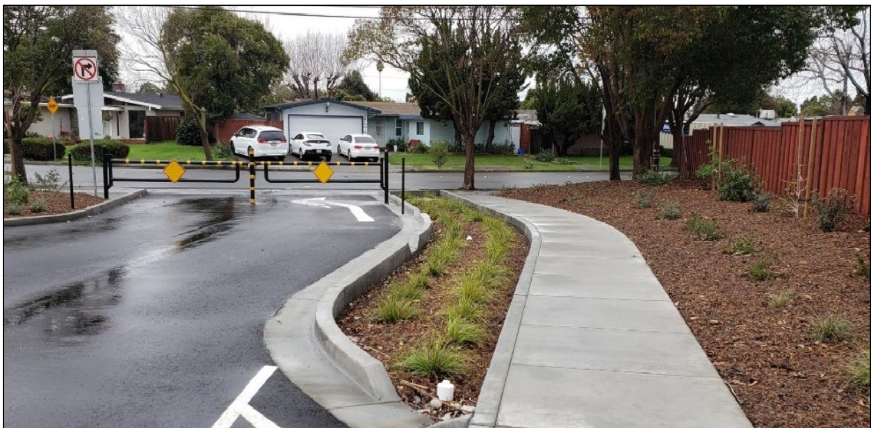
Figure B-11. Turner Court Bioretention Area. A walkway provides pedestrian access to Alameda County's Turner Court facility from the adjacent City street in the City of Hayward. The pedestrian walkway is adjacent to a bioretention area that treats stormwater runoff from the Turner Court facility's parking lot.
