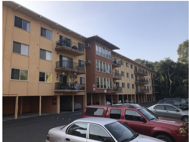
Exterior of Subject and typical tenant parking
