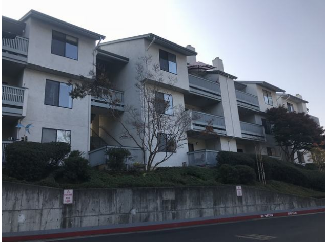
Ridgecrest Apartments north of the Subject
