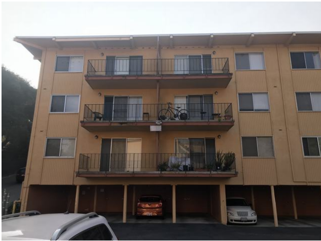
Exterior of Subject and typical tuck-under tenant parking
