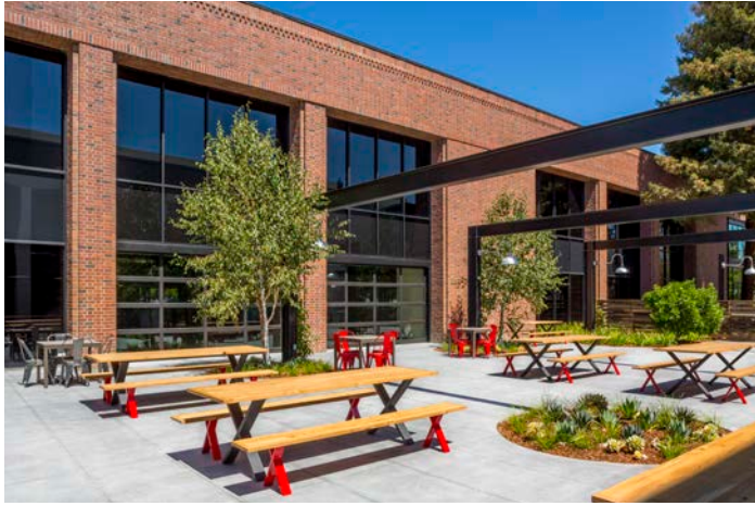
Outdoor eating area located adjacent to indoor break areas and enhanced through use of scored concrete.
