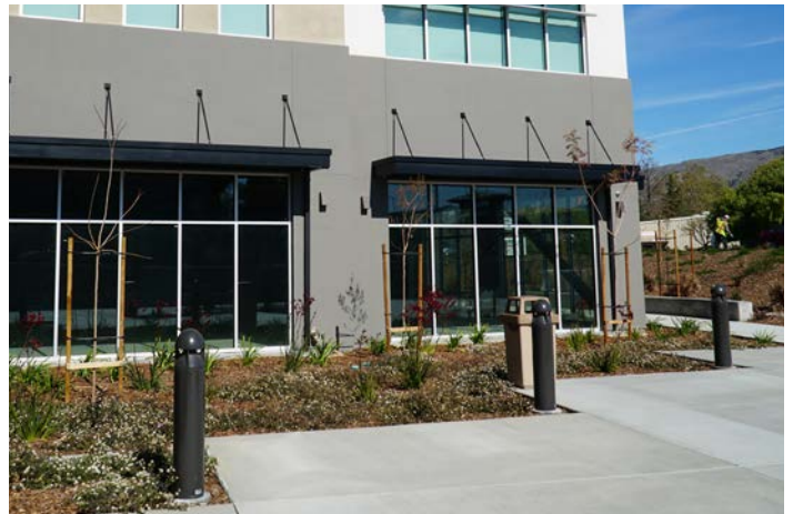
Low, bollard light fixtures placed to provide lighting within pedestrian areas.
