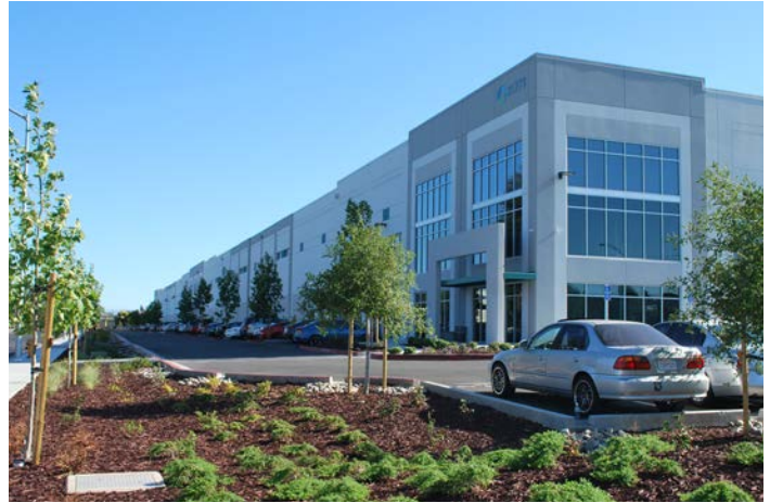
Street facing building elevation includes variation in wall plane, wall height, and roofs at different levels.
