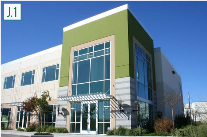
Colors, materials, trim, windows, awning, and doors provide clear identification of building entry and reinforce building design.
