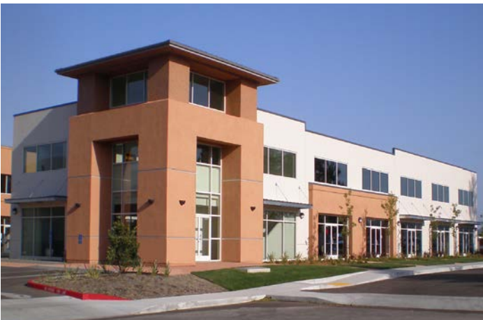
Window proportions complement architectural style and clerestory windows are used to allow interior natural daylighting.
