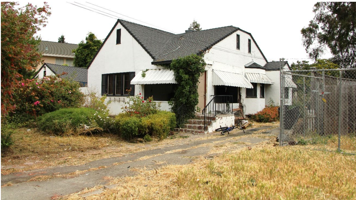
Photograph 2: View of 24656 Mohr Drive from Mohr Drive, facing northeast.
