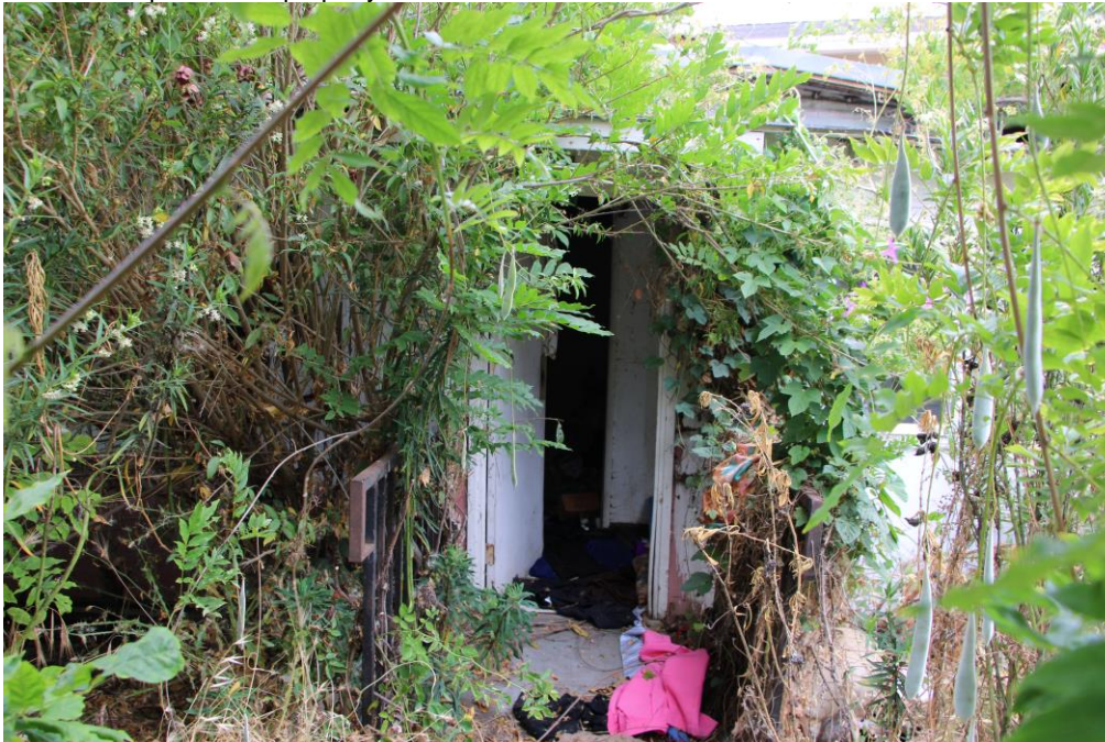
Accessory dwelling entrance with overgrowth vegetation.
