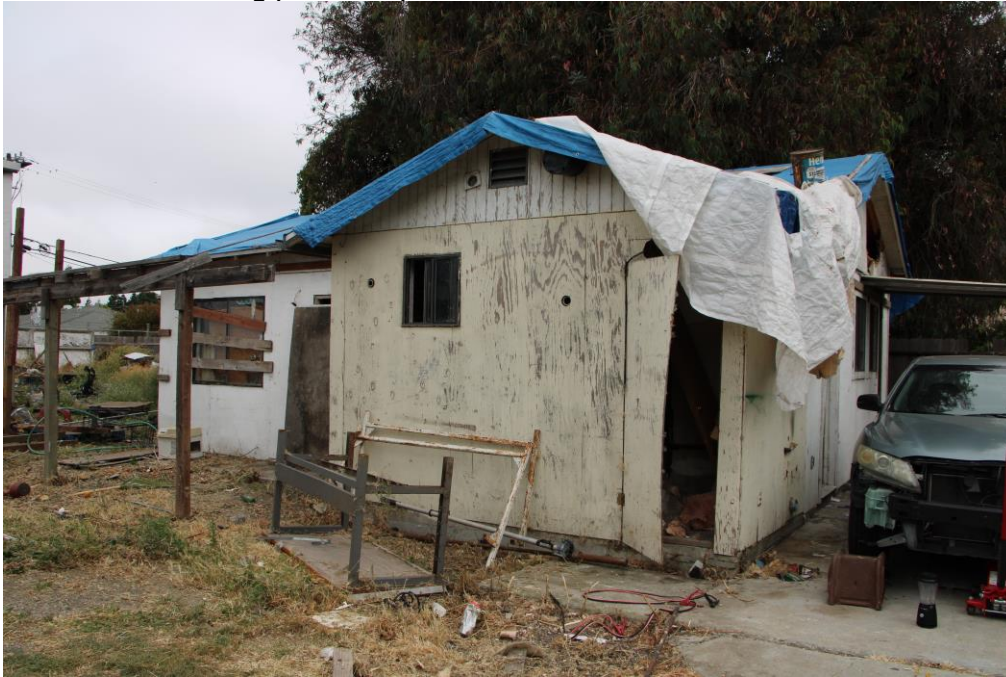
Accessory dwelling unit in rear of property.
