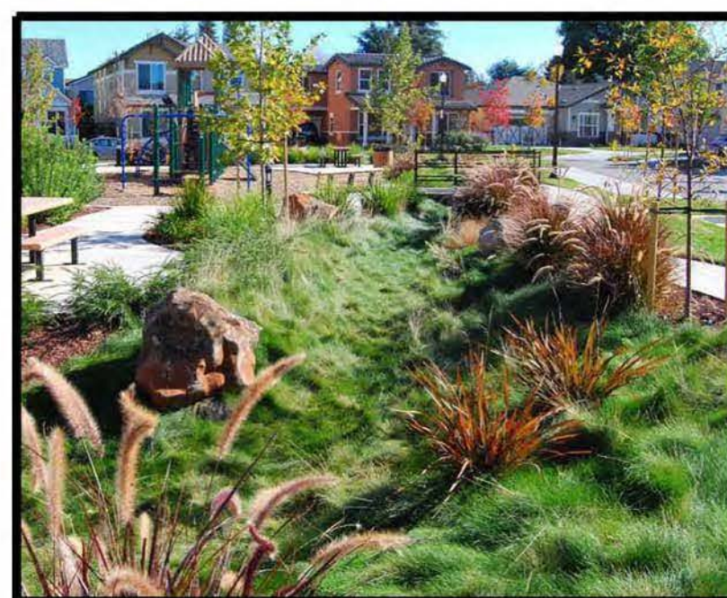
Example of Bioswale with Boulders NOTE: Grassy swale and boulders are the only items in this photo being referenced.
