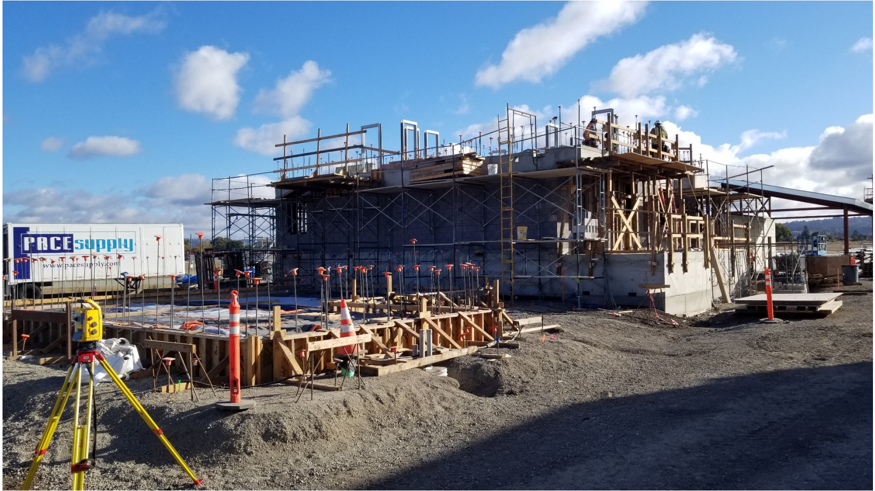
Building 4 – Storage Building & Building 5 – Burn Building (background)
