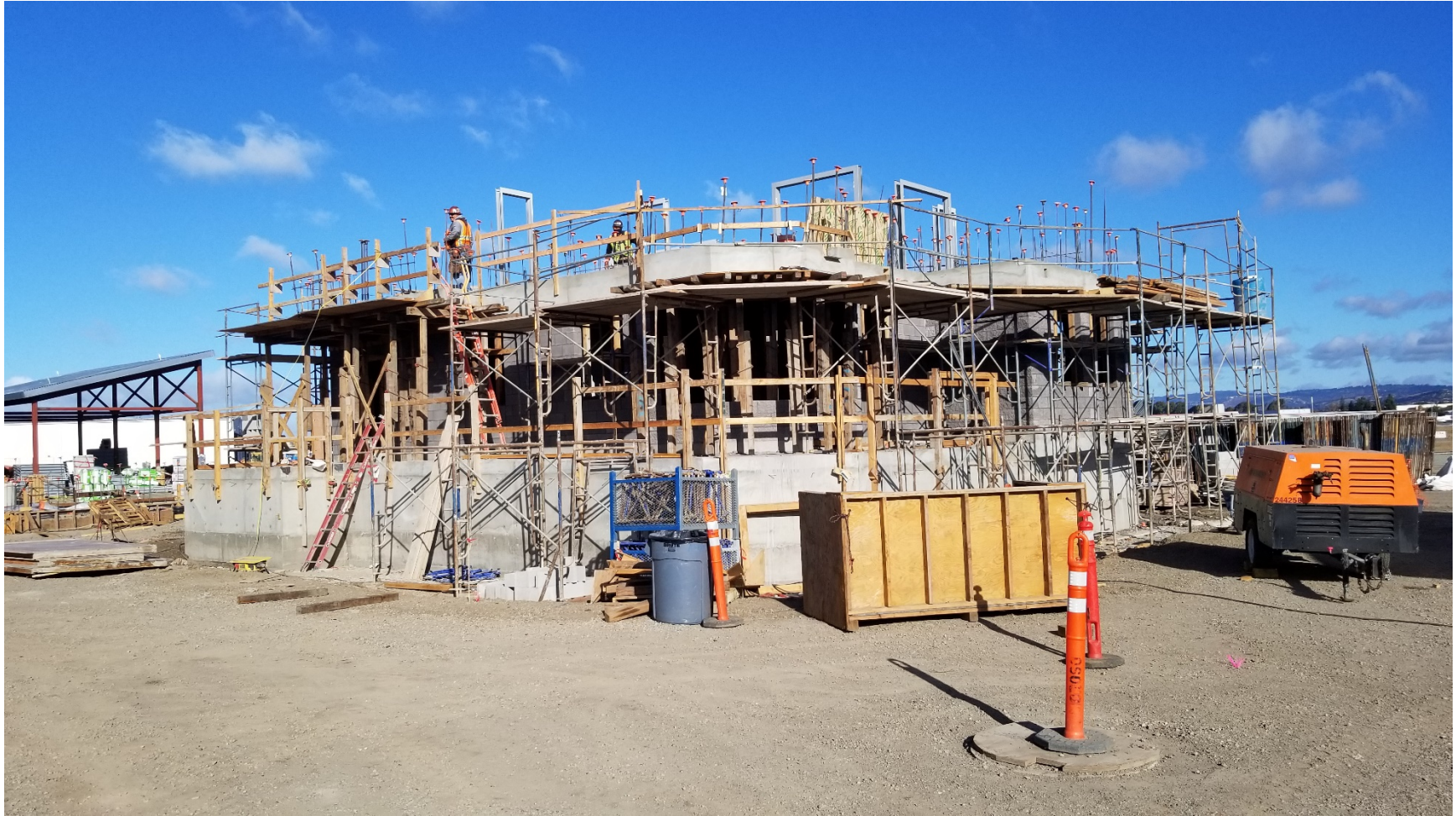
Building 5 – Burn Building
