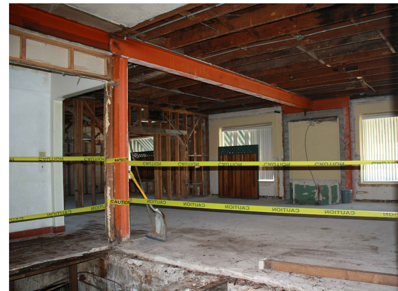
07 INTERIOR EXISTING CONDITION
