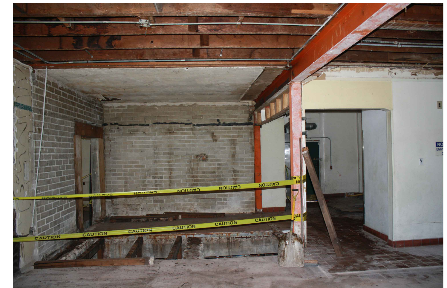
08 INTERIOR EXISTING CONDITION
