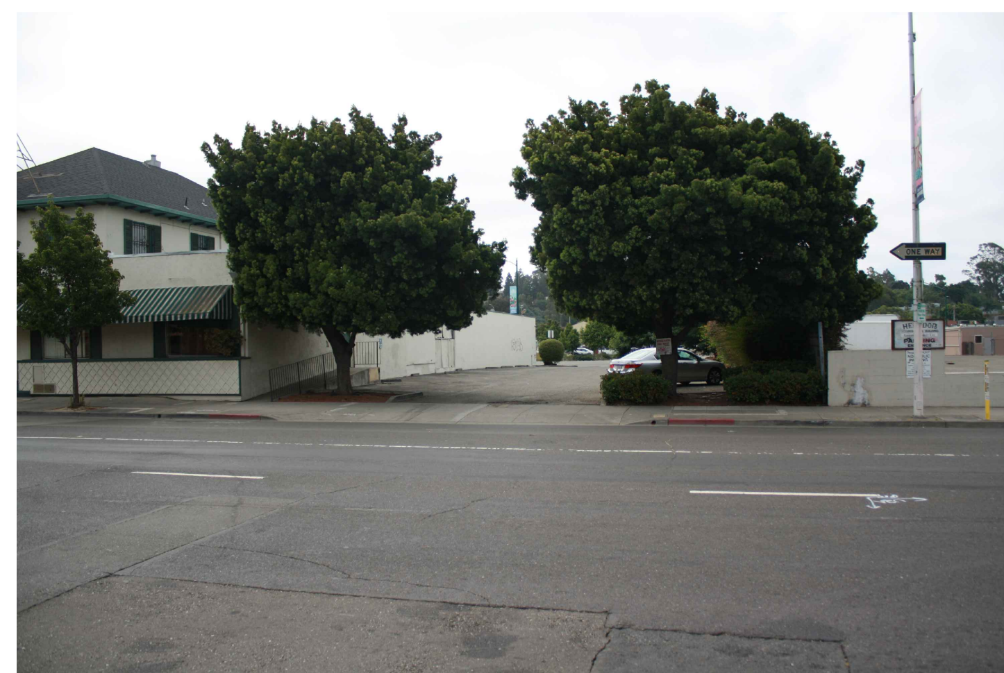
09 EXISTING BUILDING #1 'C' STREET DRIVEWAY APRON
