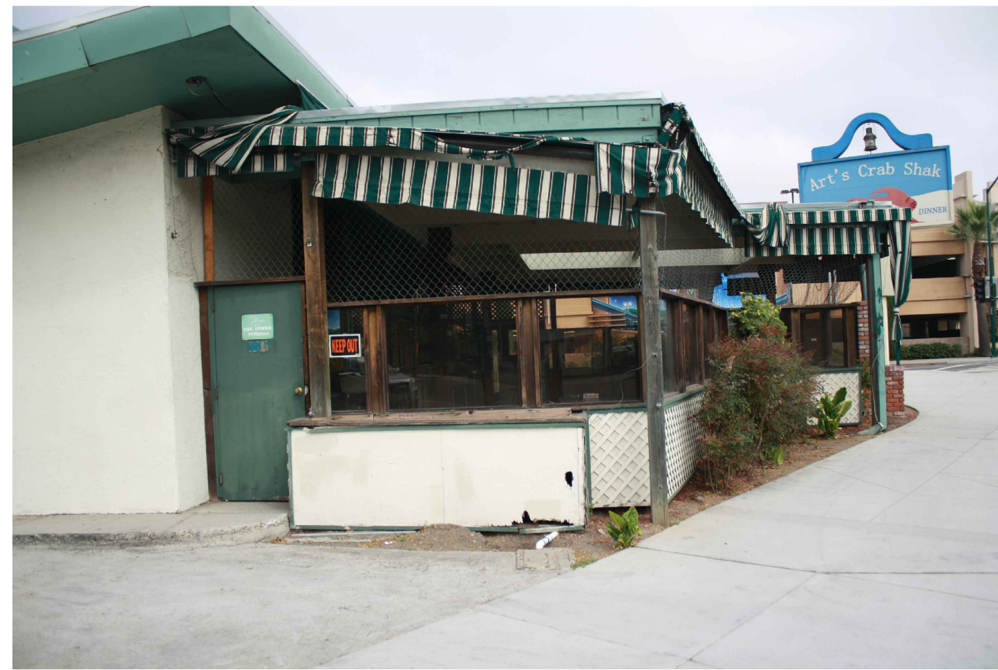
01 EXISTING OUTDOOR PATIO ENTRY
