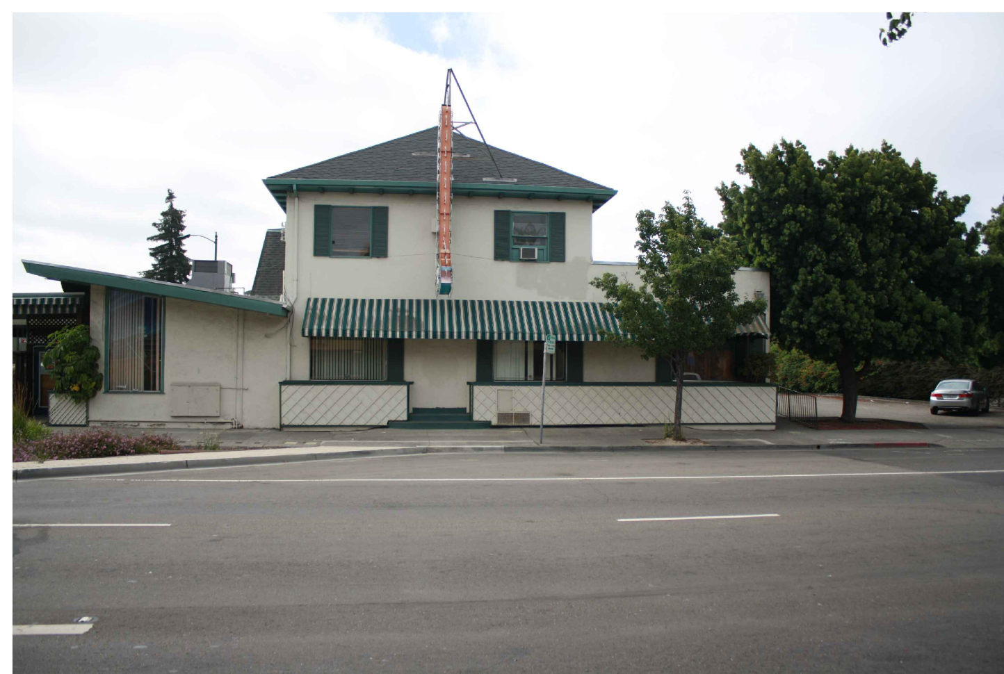
08 EXISTING BUILDING #1 FROM 'C' STREET
