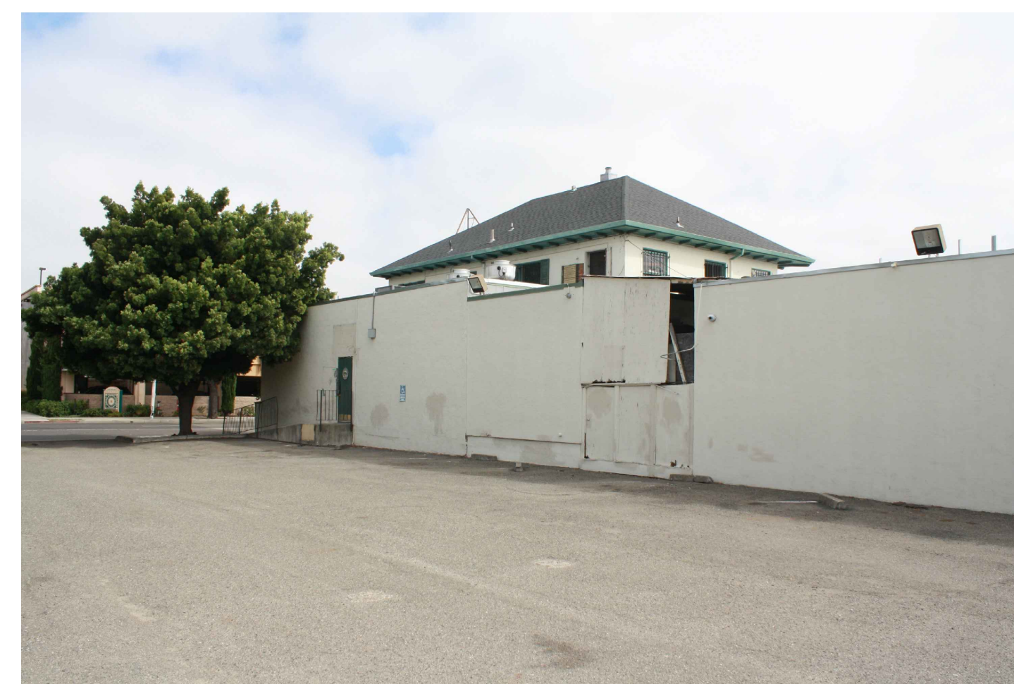
10 EXISTING BUILDING REAR ENTRY AND PARKING LOT
