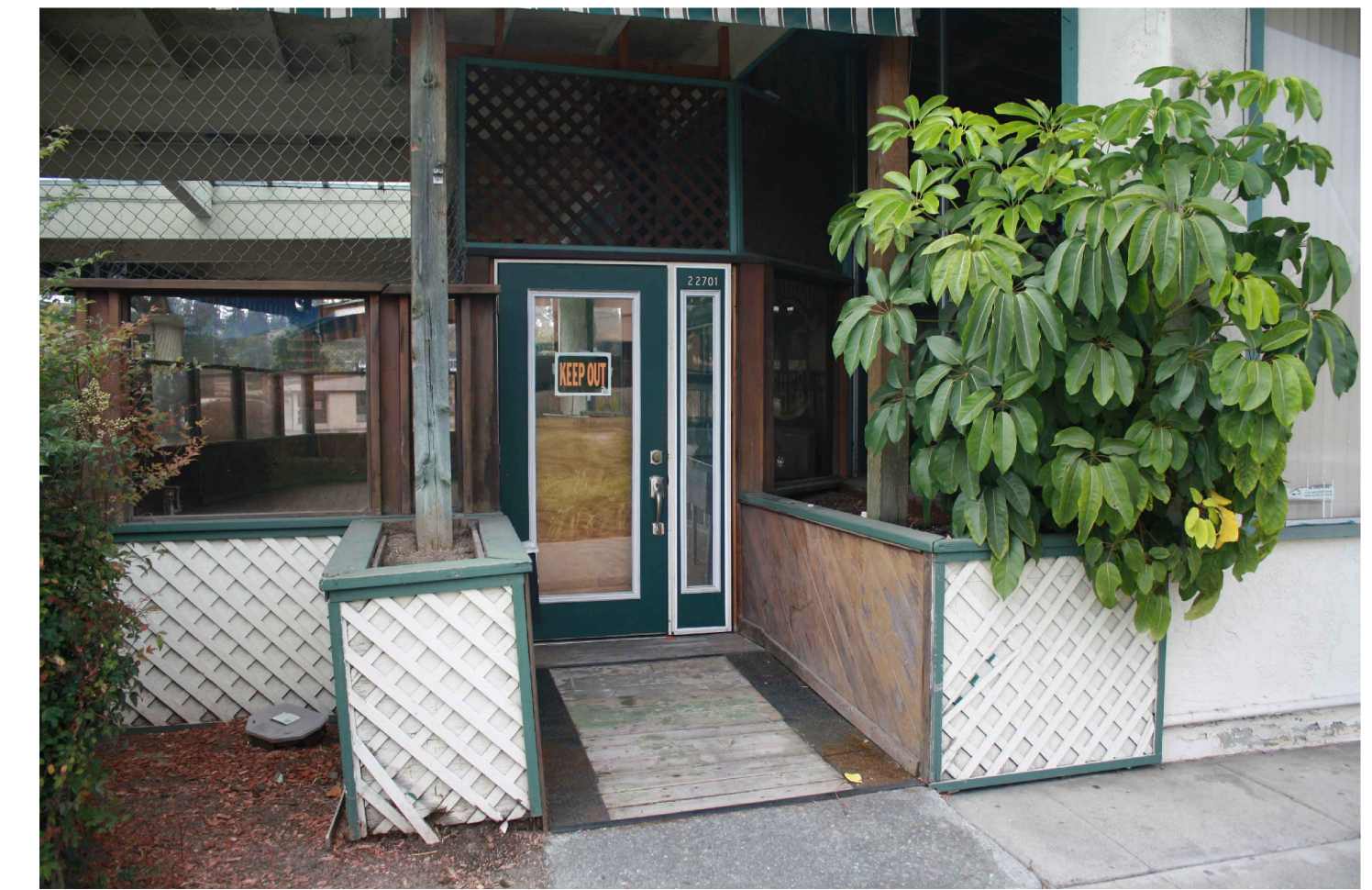
04 EXISTING OUTDOOR PATIO ENTRY
