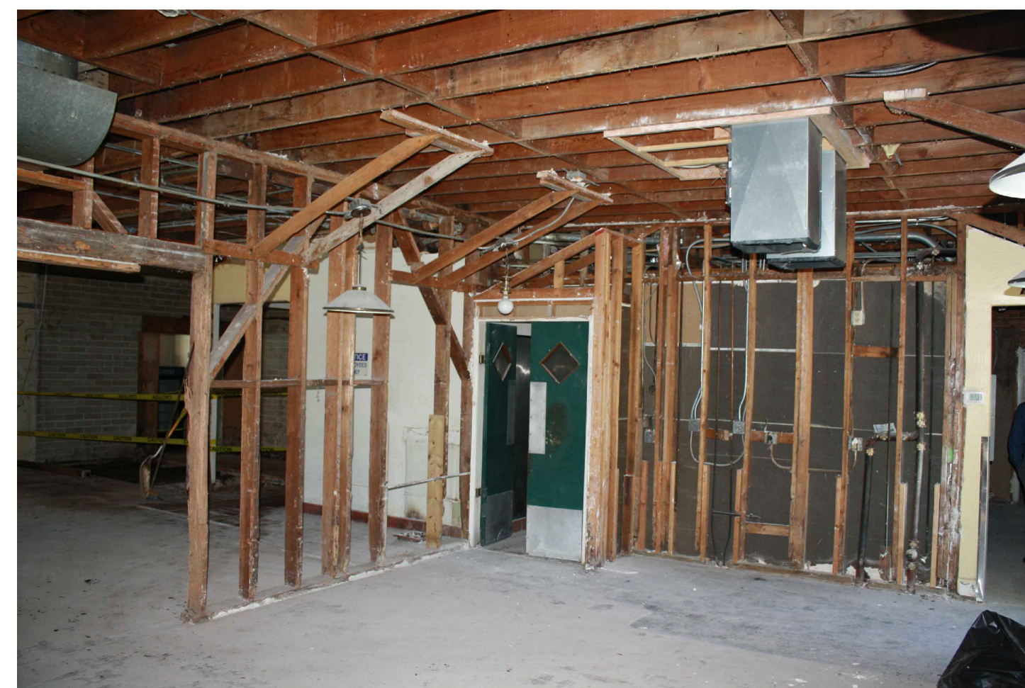
10 INTERIOR EXISTING CONDITION
