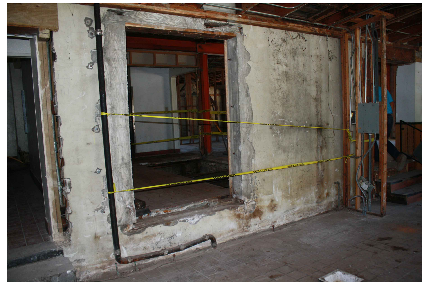
06 INTERIOR EXISTING CONDITION
