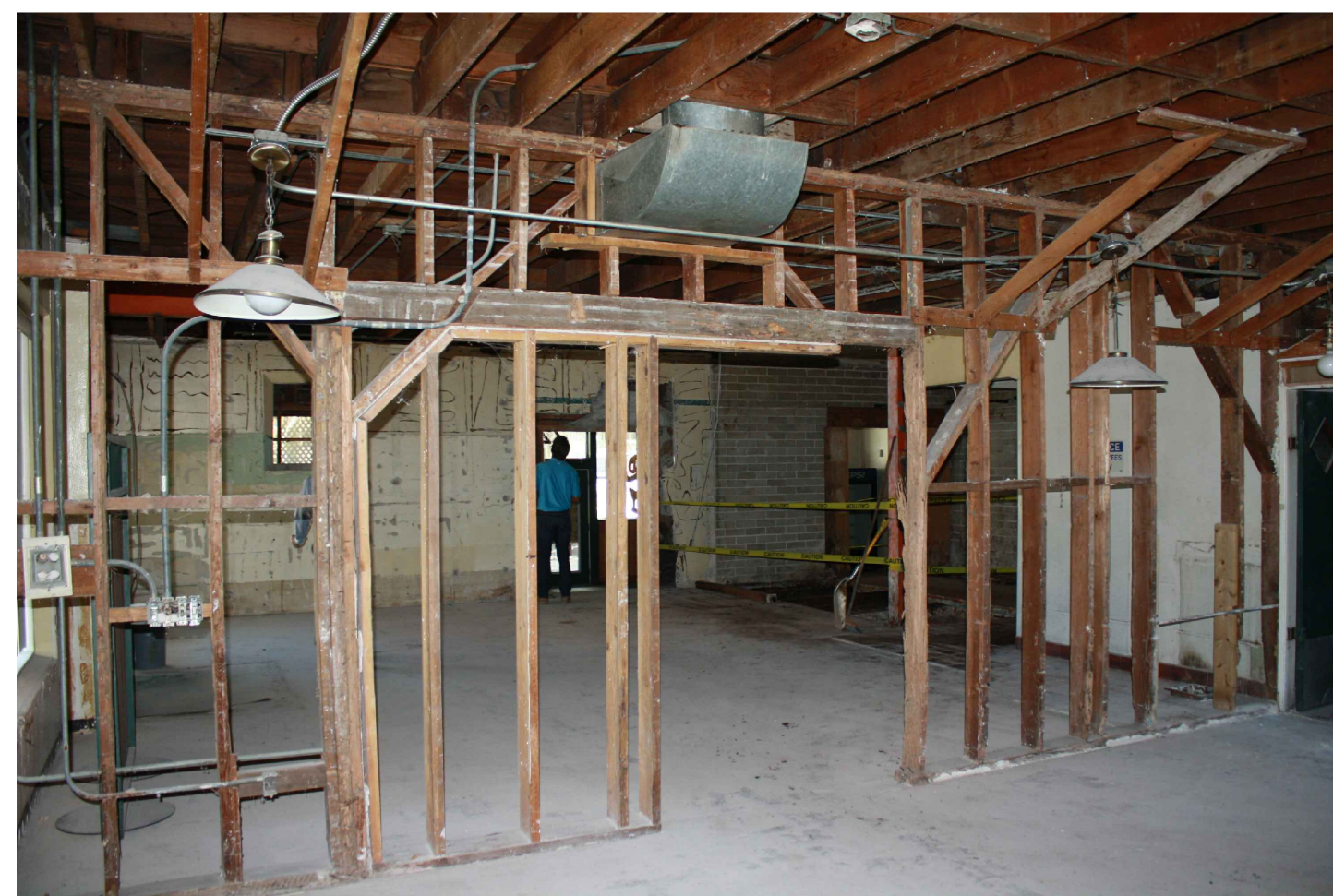
09 INTERIOR EXISTING CONDITION
