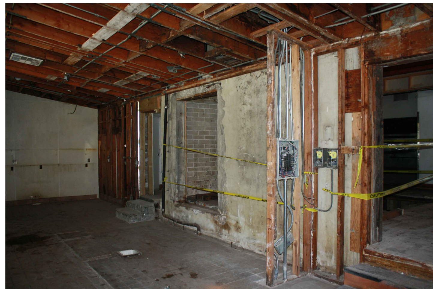
05 INTERIOR EXISTING CONDITION
