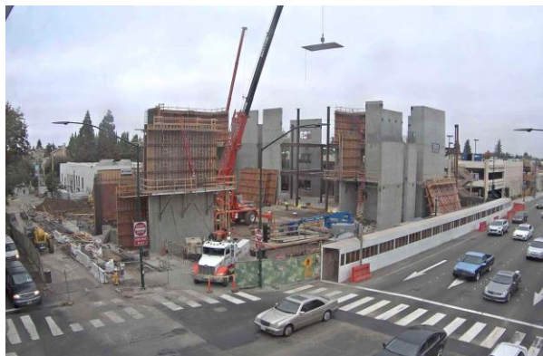
Photo of construction progress, Sept 16, 2016
