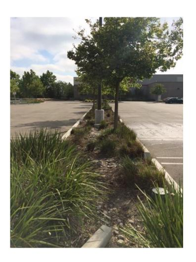
Bioswales for Stormwater Treatment
