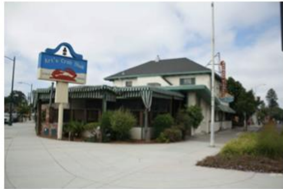
07 EXISTING BUILDING #1 CLOSEUP
