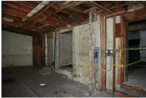
05 INTERIOR EXISTING CONDITION
