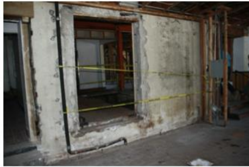
06 INTERIOR EXISTING CONDITION
