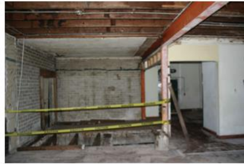
08 INTERIOR EXISTING CONDITION
