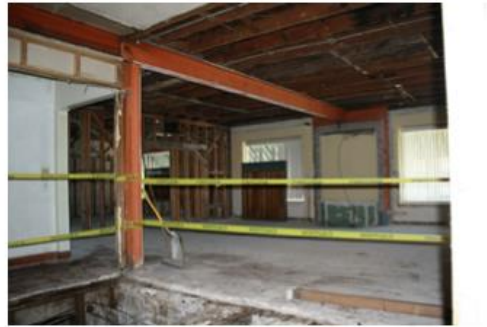
07 INTERIOR EXISTING CONDITION
