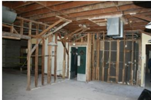
10 INTERIOR EXISTING CONDITION
