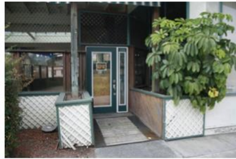
04 EXISTING OUTDOOR PATIO ENTRY
