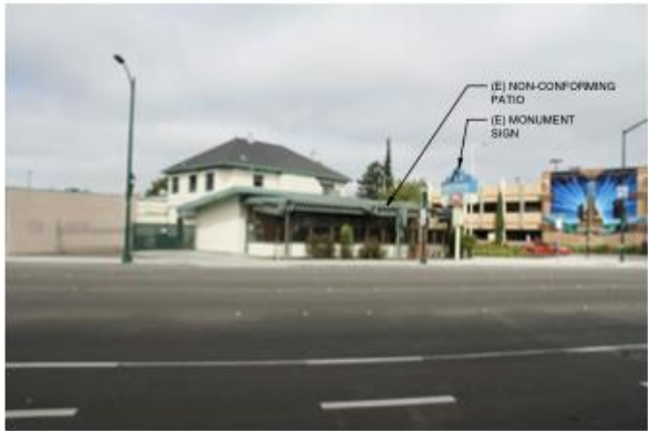
05 EXISTING BUILDING #1 AND ADJACENT PARKING STRUCTURE
