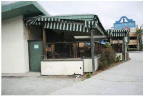
01 EXISTING OUTDOOR PATIO ENTRY
