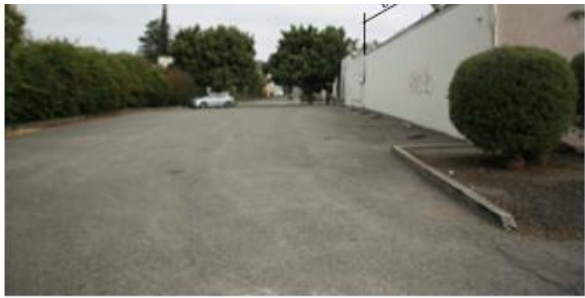
01 EXISTING PARKING LOT
