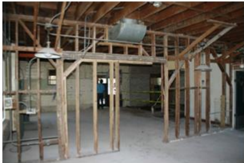
09 INTERIOR EXISTING CONDITION
