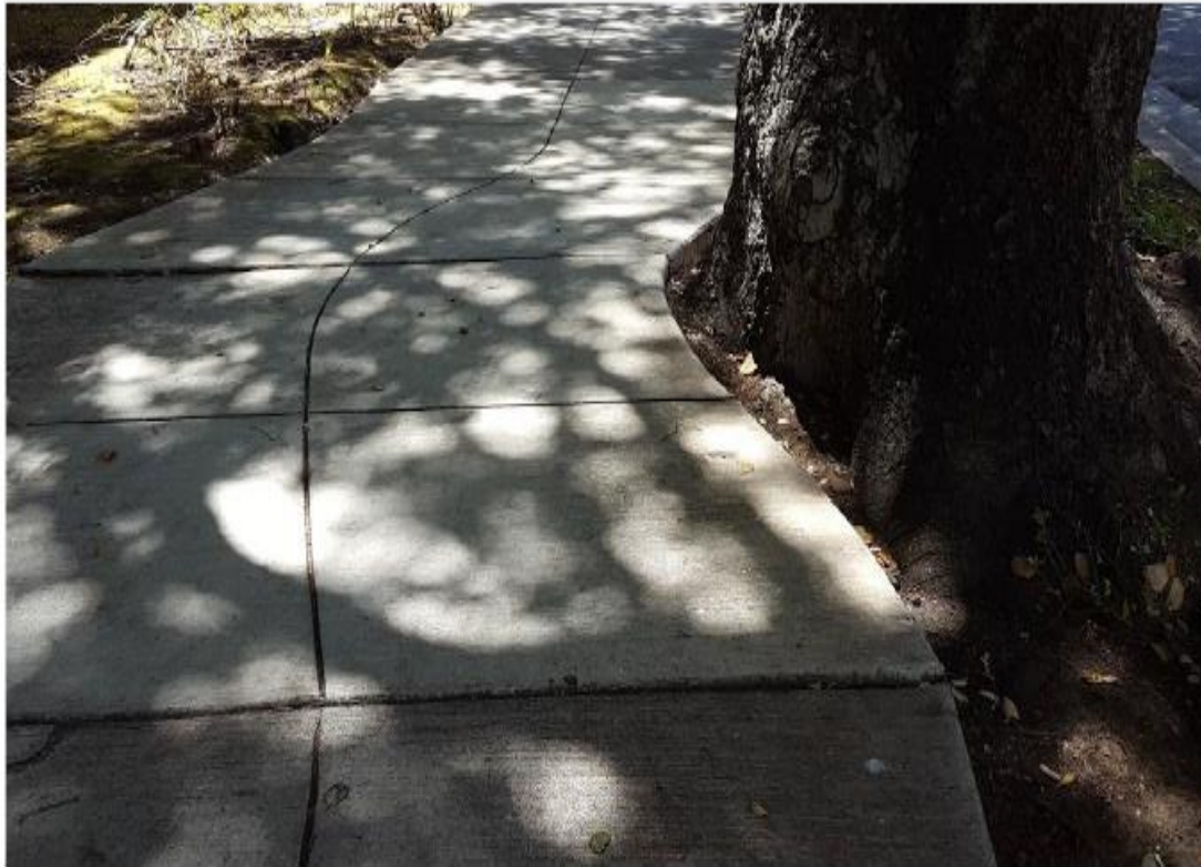
Figure 11. City curved the sidewalk around the mature oak's trunk to provide extra space (Palo Alto).
