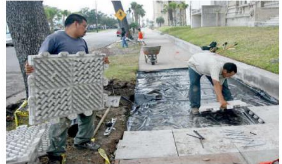
Figure 31. Photo of Terrewalks® installation in Galveston, Texas.
