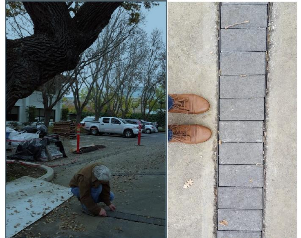
Figure 35. Root path installation radiating out into parking lot to improve the root zone of a high-value tree (Palo Alto).
