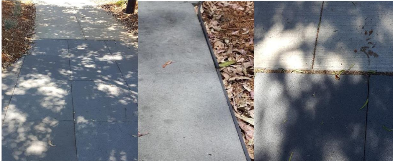
Figure 29. Close-up view of rubber sidewalk installation (University Circle, Palo Alto 2016).
