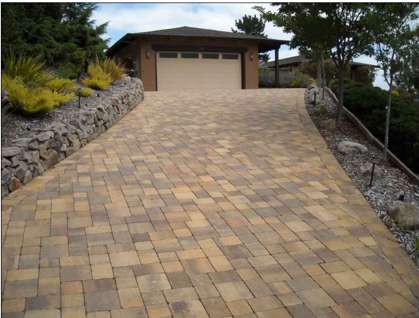
E DRIVEWAY CONCRETE PAVERS NTS
