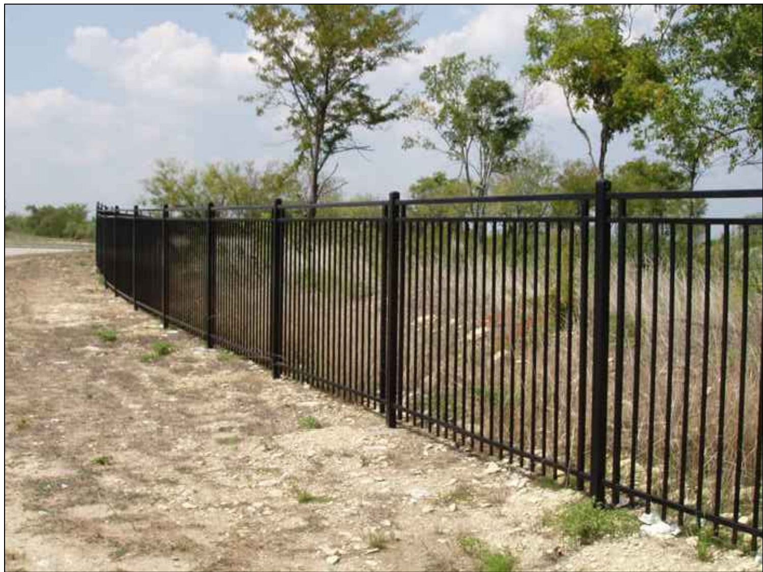
A 6' WROUGHT IRON PERIMETER FENCE NTS
