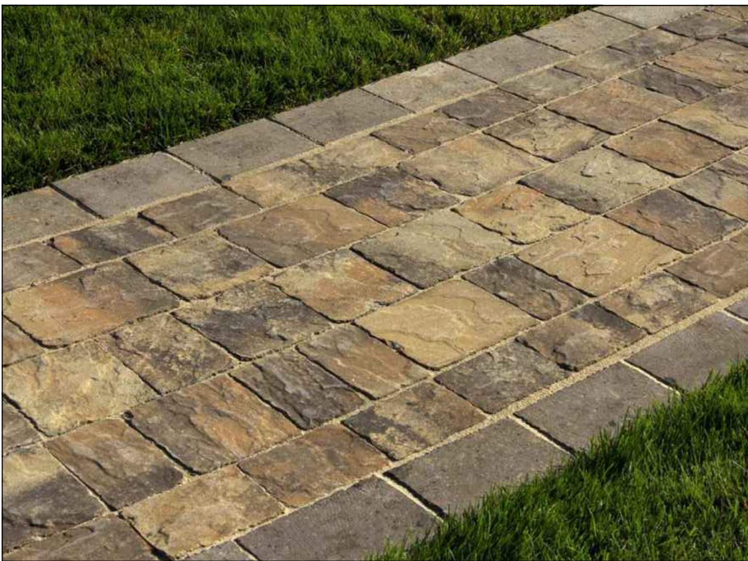
F FRONT WALK CONCRETE PAVERS NTS
