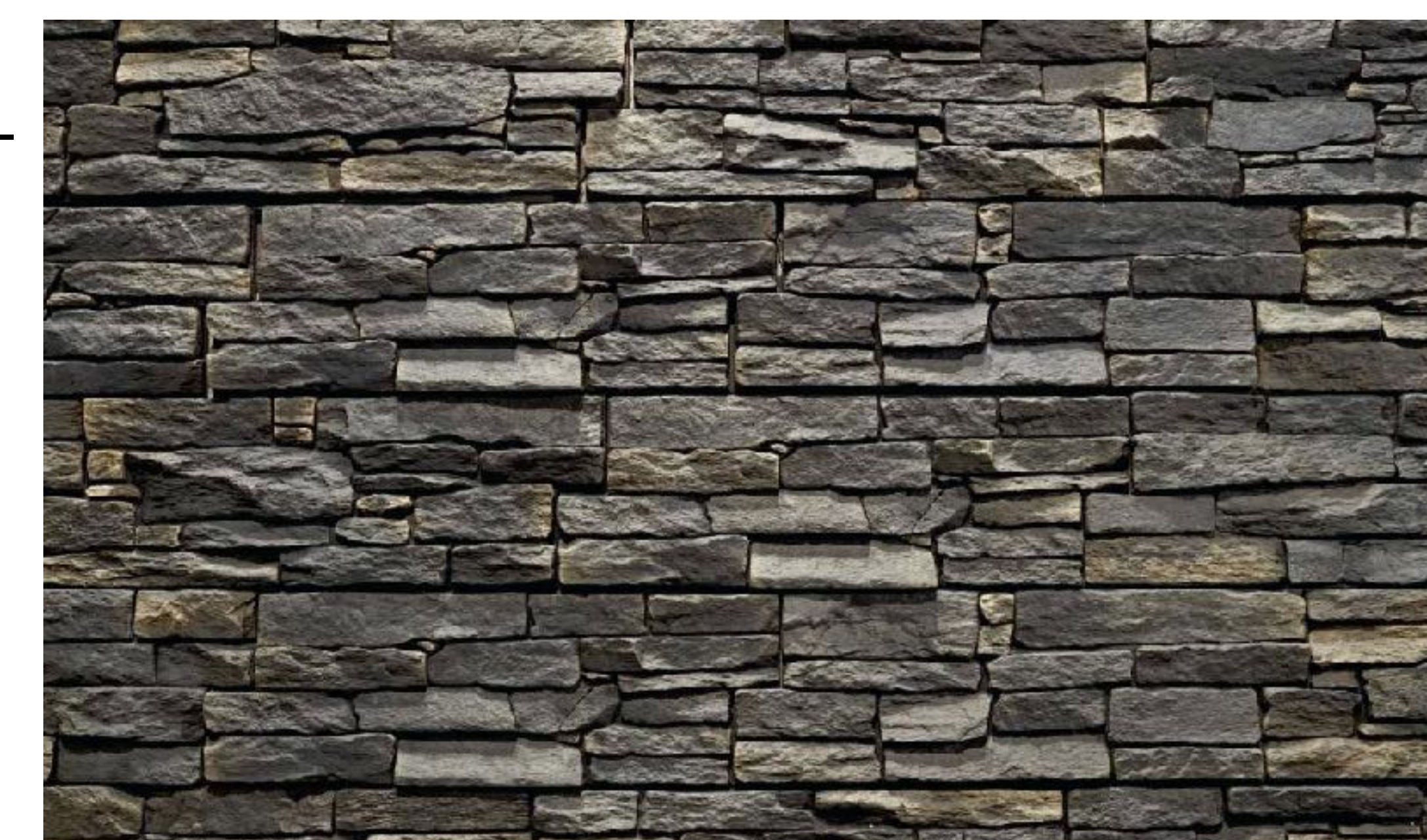
DRY STACKED STONE WAINSCOTING
