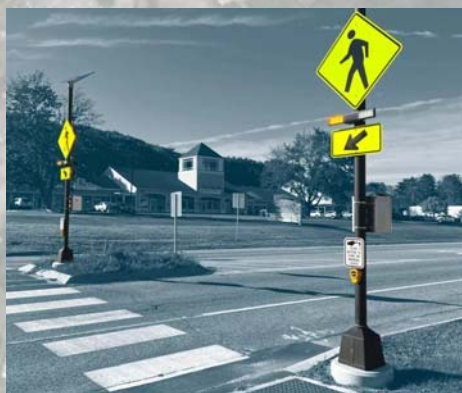
Rectangular Rapid Flashing Beacon
