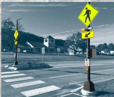
Rectangular Rapid Flashing Beacon
