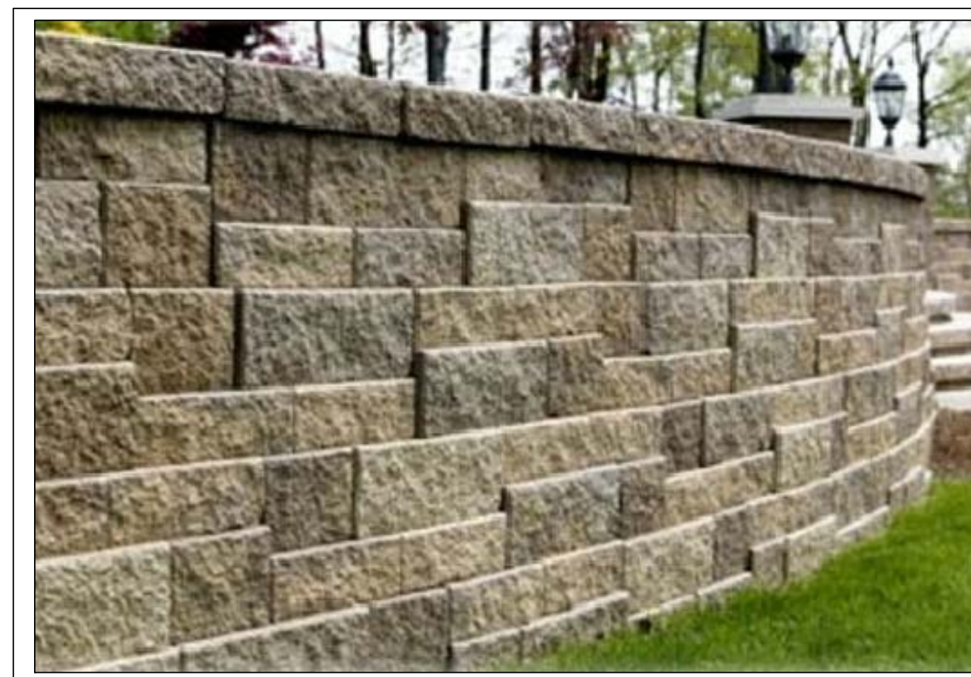
RETAINING WALL WITHIN BIO-RETENTION BASIN (VERA-LOK, MOSAIC BLOCK, ALLEGHENY BLEND COLOR)
