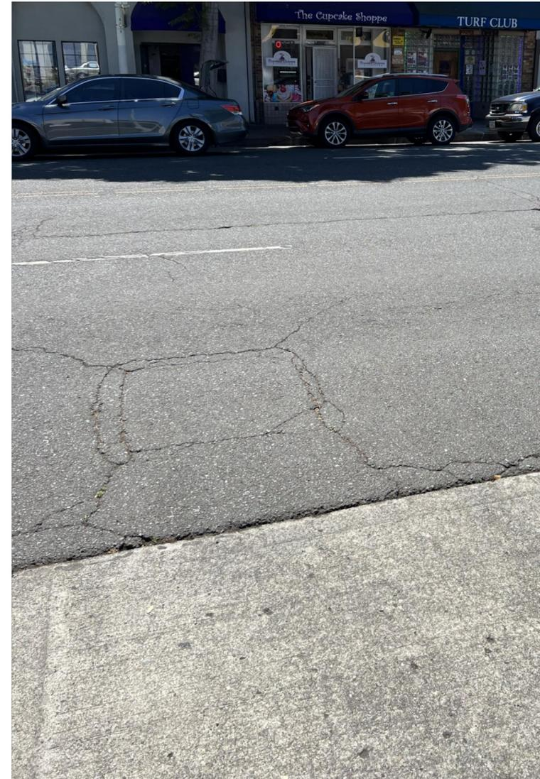
Tree root damage to sidewalk
