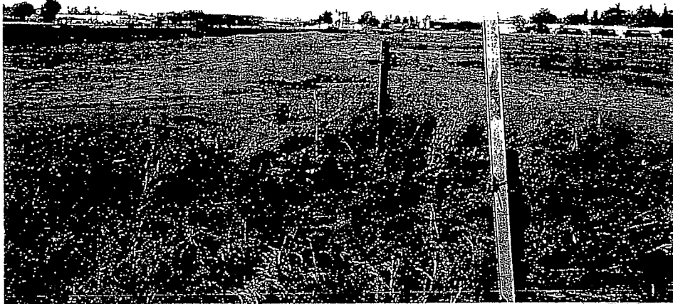
Photograph 7: Signposts for natural gas transmission line. Northern portion of site, view to north.
