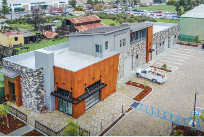
Unique paving at driveway highlights site entry while building is oriented to allow for daylighting of interior work areas.
