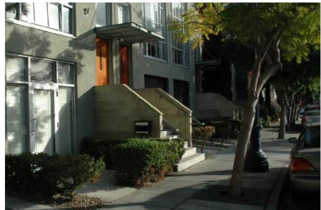
Stoop with paired entries to dwelling portion of Live/Work units.
