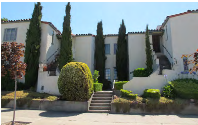
2-story Courtyard building.
