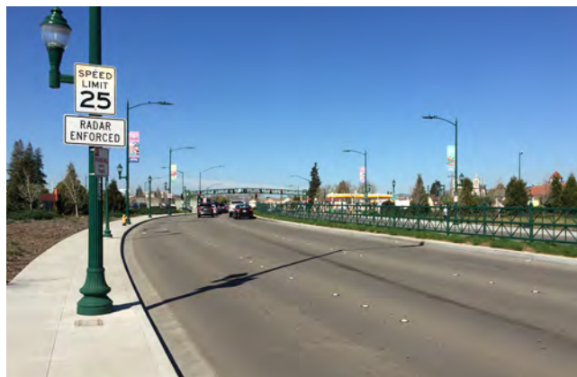
Sidewalk along Foothill Boulevard north of Mission Boulevard
