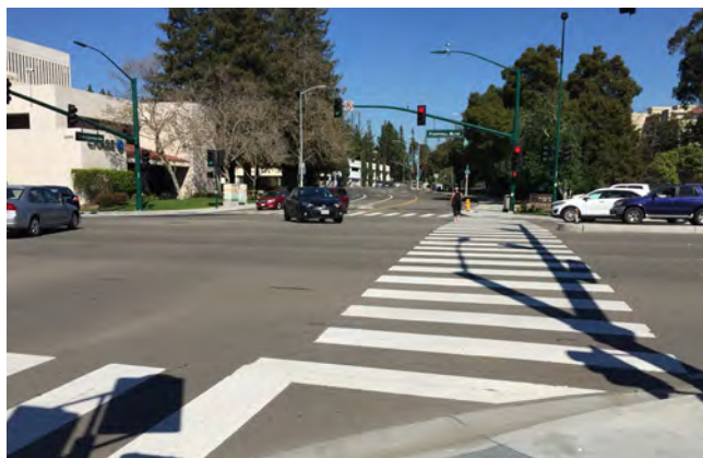
Crosswalk on Foothill Boulevard at City Center Drive
