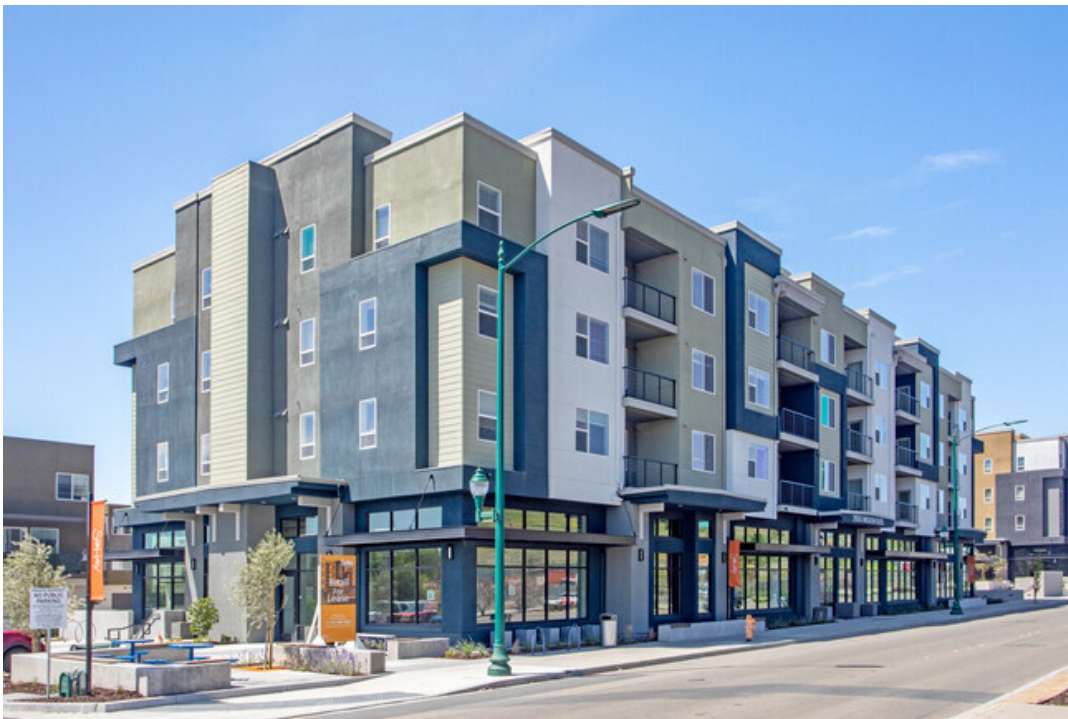
The Mix / Hayward, CA. Building height to the highest roof plane is 46' for 4 stories and to the highest parapet is 55'
