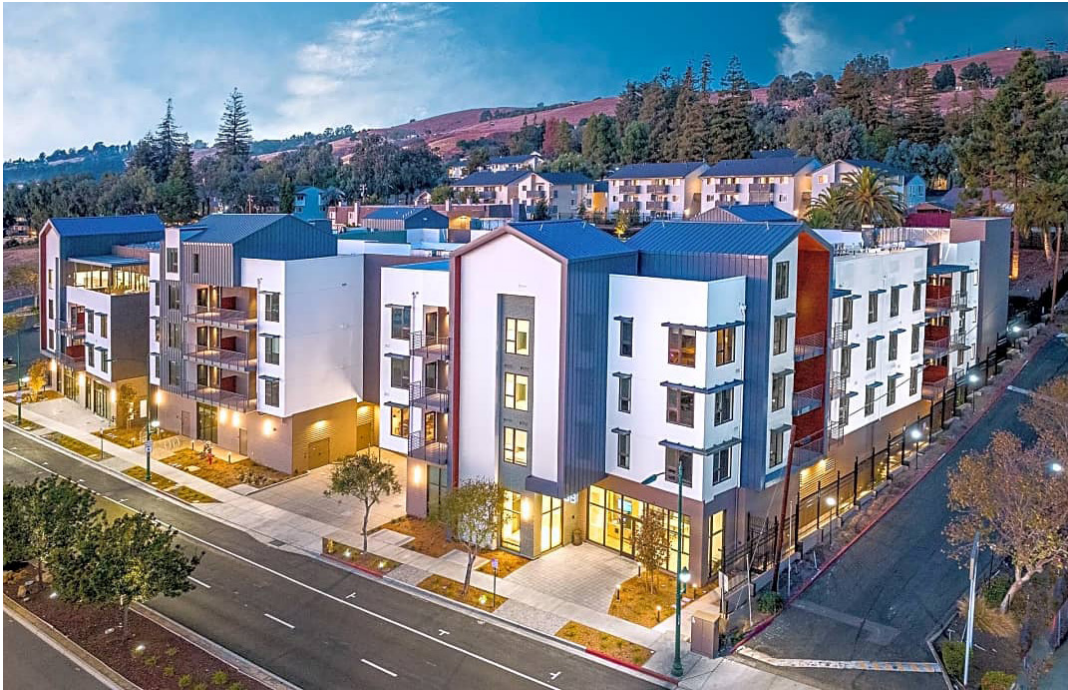
Legacy / Hayward, CA. Building height is about 44 feet for 4 stories, with an allowance for some areas to be taller than 44 feet to accommodate architectural elements.
