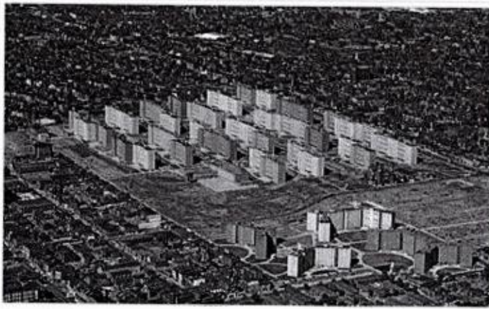
The Pruitt-Igoe complex (demolished as from 1972 to 1976) was composed of 33 buildings of 11 stories each, located on 57 acres [5] of the Near North Side of St. Louis, Missouri. The four large branching structures in the foreground were the Vaughan Public Housing Complex (also demolished). Also pictured is the Pruitt School (the four-story building near the center of the photo) and St. Stanislaus Kostka Church, both of which still stand.
