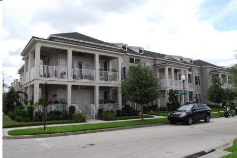
Rowhouses with 2-story porches massed as one building.
