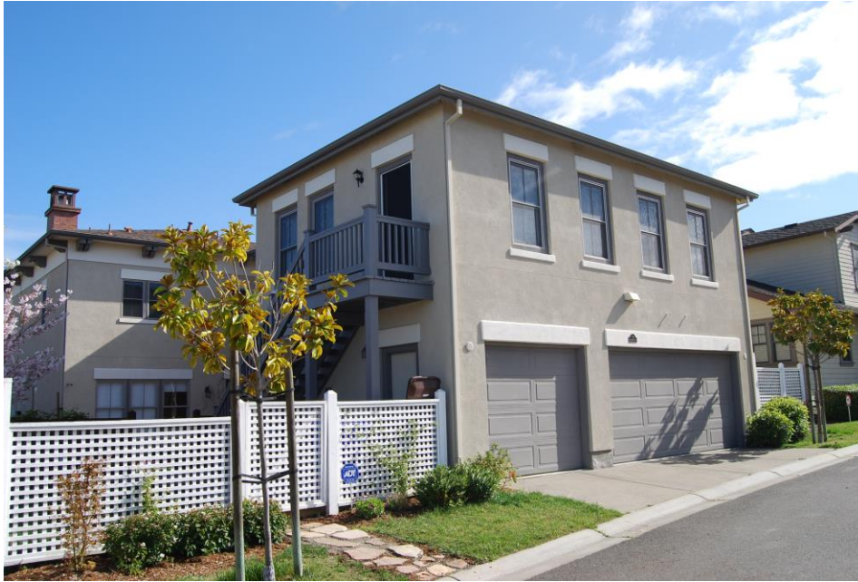
Two-story Carriage Building with living unit above
