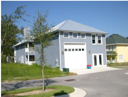
Two-story Carriage Building with living unit above
