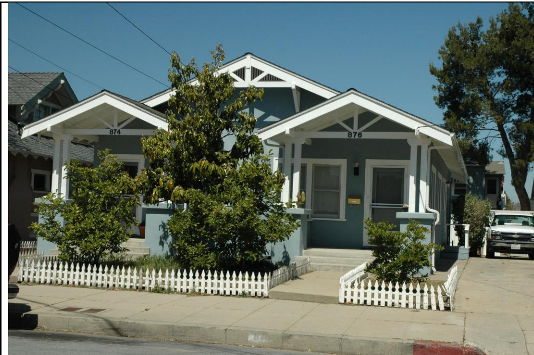
Duplex side-by-side units, each with projecting porch.
