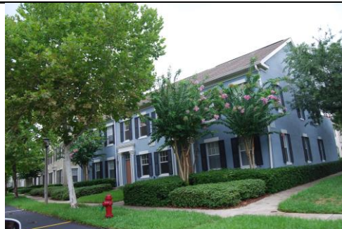
2-story Multiplex Large with front yard.
