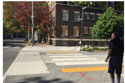
Example of at-grade crossing at shared street intersection, in Seattle, WA
