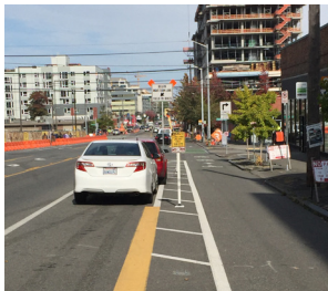
Class IV Protected Bike Lane adjacent to on-street parking
