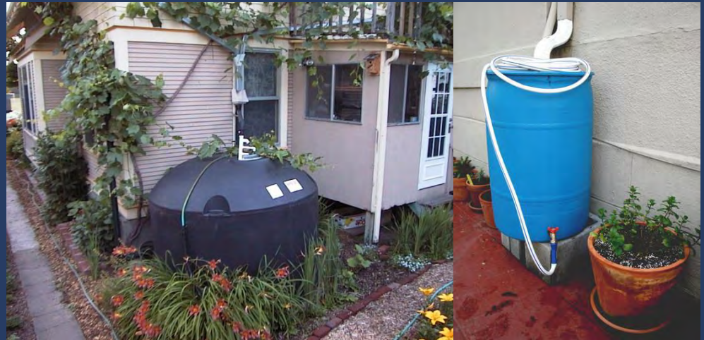
Rainwater Harvesting (approximately 250 and 50-gallon barrels)
