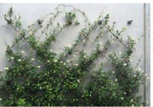
Vertical wire trellis system installed on facade of existing medical building to utilize small planting strip for vine growth.
