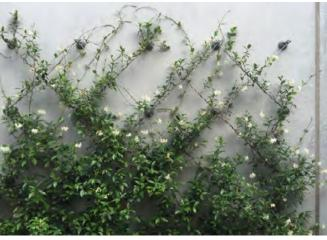
Vertical wire trellis system installed on facade of existing medical building to utilize small planting strip for vine growth.
