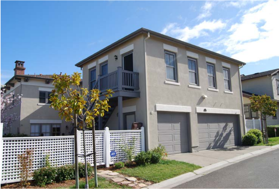
Two-story Carriage Building with living unit above
