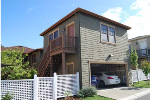
Two-story Carriage Building with small living unit above
