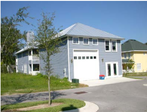
Two-story Carriage Building with living unit above
