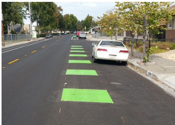
BROKEN GREEN BIKE LANE
